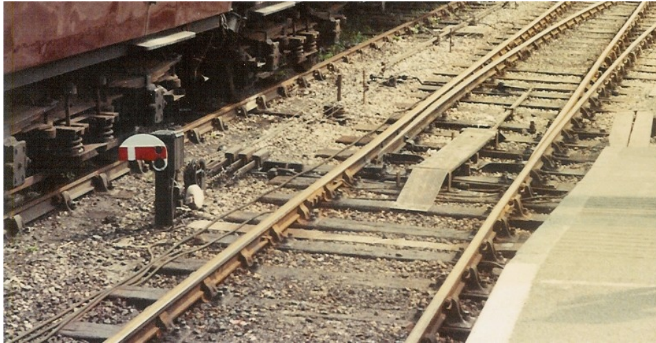
Figure 16A. A point with three detectors. The point seems to be operated by an "economic lock" entering from the crossing end of the point and with no detector bar. (Taken c.2000 Midland Railway Centre)
