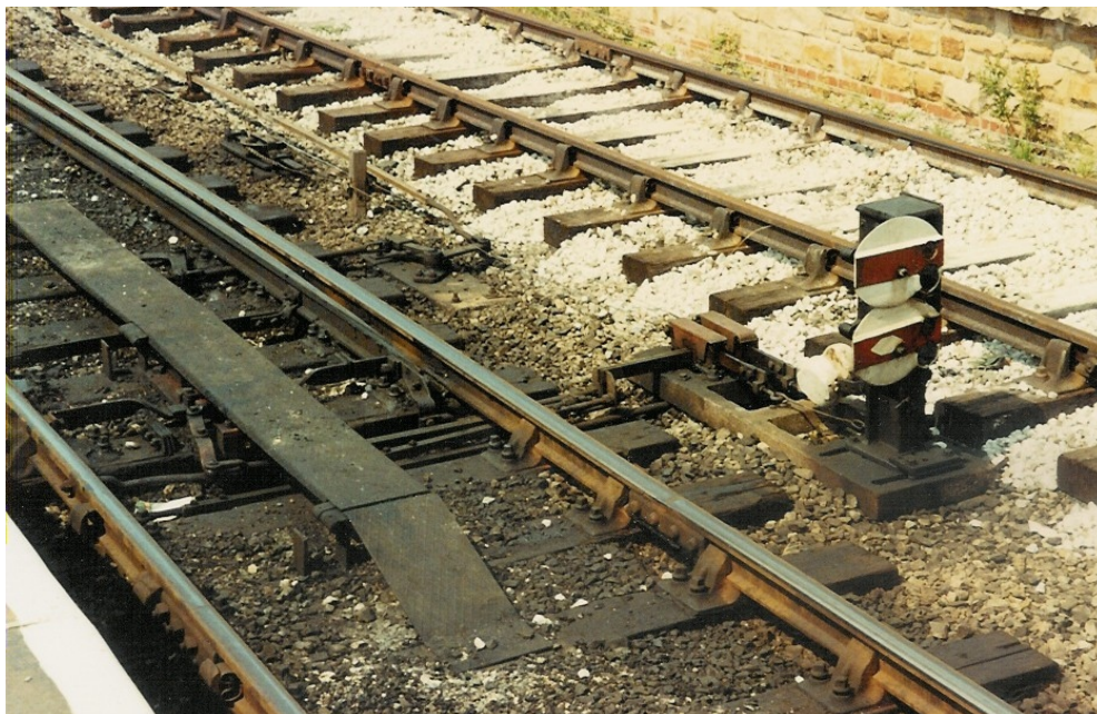
Figure 16C. Stretcher bars, detectors and operating rods and a narrow cover obscuring the point operating mechanism (taken c.2000) at Midland Railway Centre.
